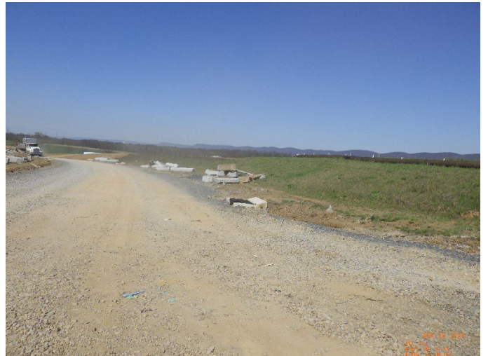
4. Existing curbs and utilities being removed.
