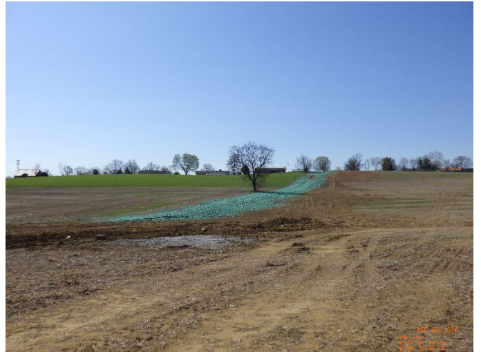
2. Active waterline installation and stabilization.
