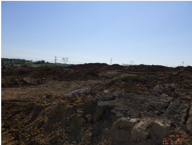
3. Active drilling and blasting.
