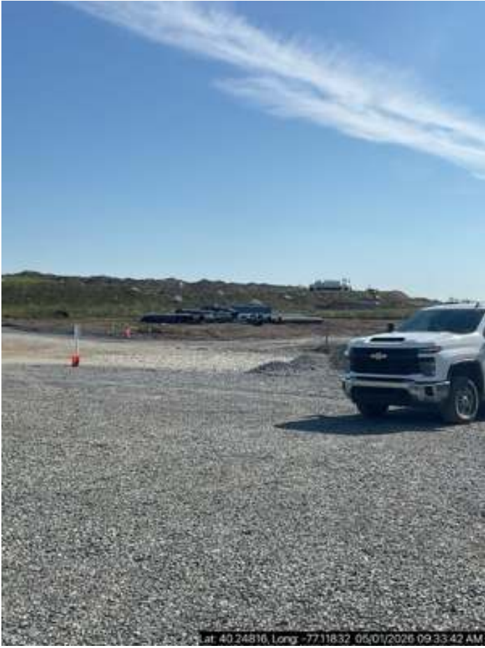
1 - Loading of a blast on date of this inspection.
