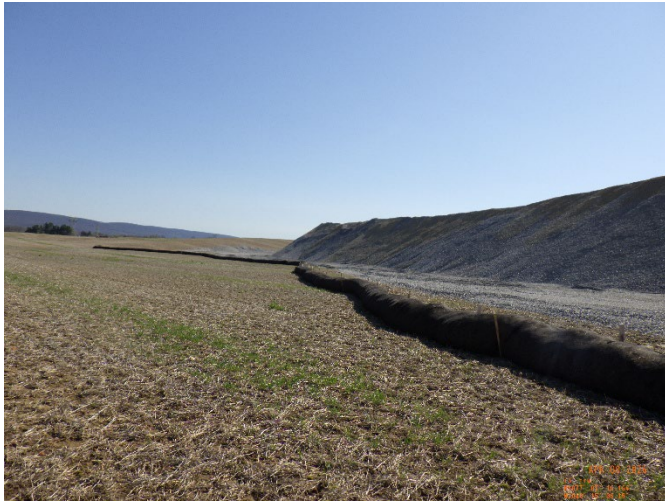
1. Stone stockpile protected with compost filter sock.
