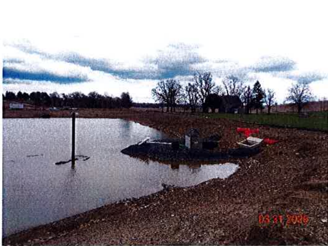
1. Trash rack and skimmer with stone landing berm installed in Sediment Basin A.
